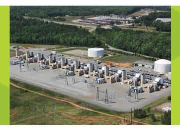
Plant Dahlberg is a natural gas-fueled, simple-cycle combustion turbine electricgenerating plant located near Commerce, Georgia, in Jackson County. The plant is used to generate electricity for South – the fastest growing region in the country. Eight of the ten units went online in 2000, while the other two went online in 2001.
