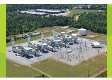
Plant Addison is a natural gas-fueled, simple-cycle combustion turbine electricgenerating plant located near Thomaston, Georgia in Upson County. The plant is used to generate electricity for the South – the fastest growing region in the country. The four units went online in June 2000.
